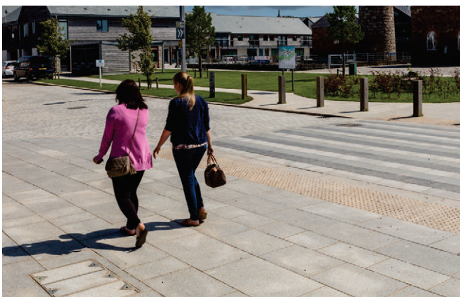
Figure 2.20: Example of the use of high quality materials to provide a safe, accessible and attractive at-grade junction crossing
